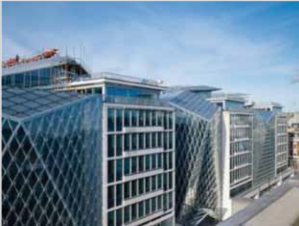
55 Baker Street: external frontage
